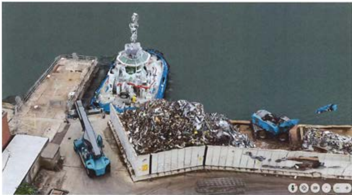
Figure 24: Access and infrastructure issues at Berth 46 Nib
