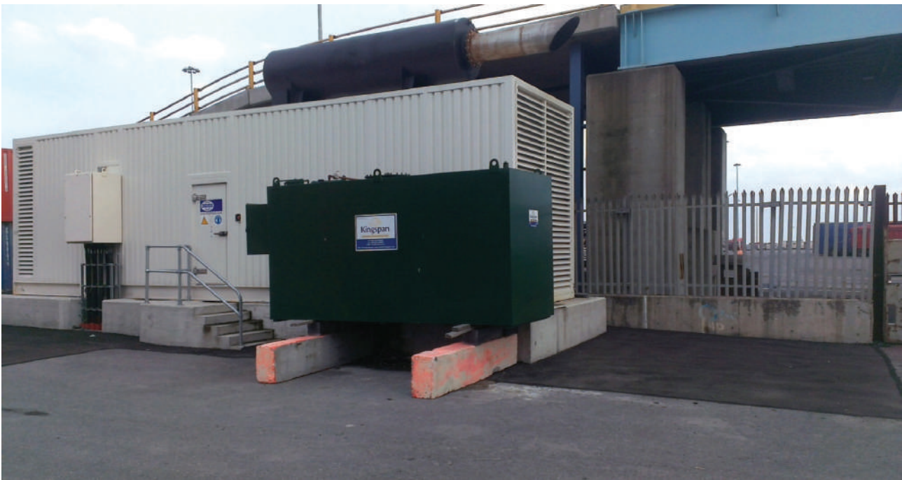
New Emergency 2.5 Mega Watt Back-up Generator.
