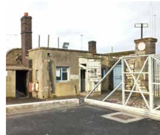
▲ View from Docks' Site looking north-west towards former Dock Gate Keeper's Hut
