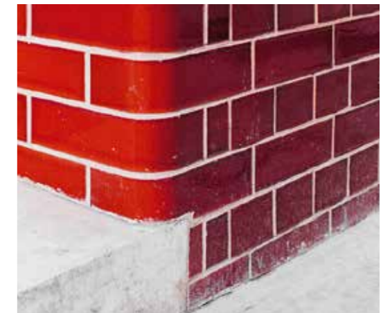
▲ Reference Image of Glazed Red Brick Wall
