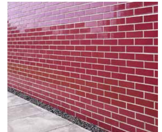
▲ Reference Image of Glazed Red Brick Wall
