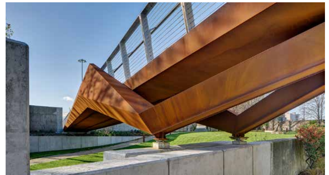
▼ Bridge - Pedestrian walkway designed as a cantilever to land lightly on the existing podium making use of existing concrete Moat walls
