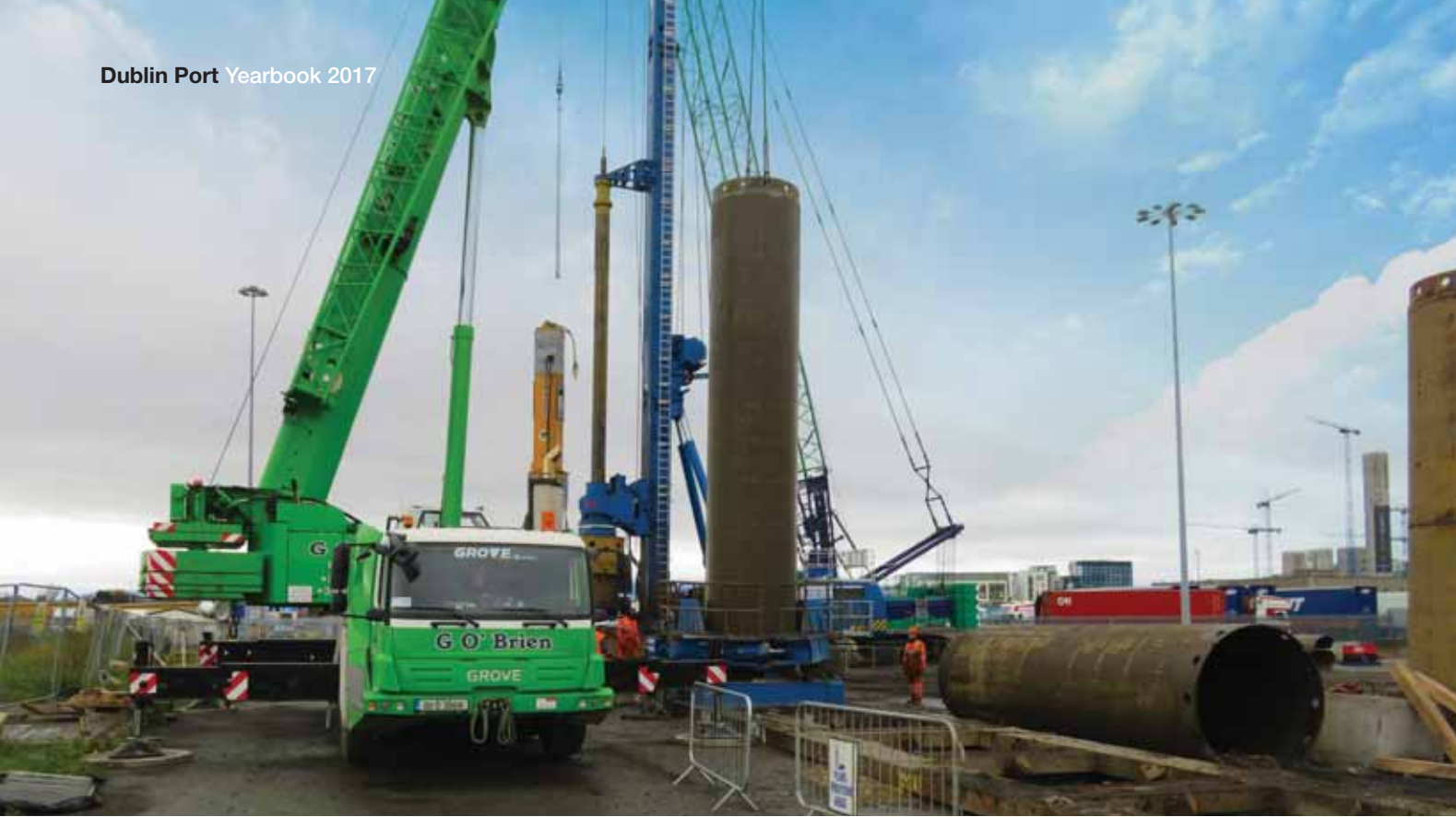
Cross Berth Quay, at the western edge of Alexandra Basin, is the location for one of the largest piling rigs in Ireland, which has begun inserting steel piles that are 35 metres long and 1.4 metres in diameter into the sea bed.
