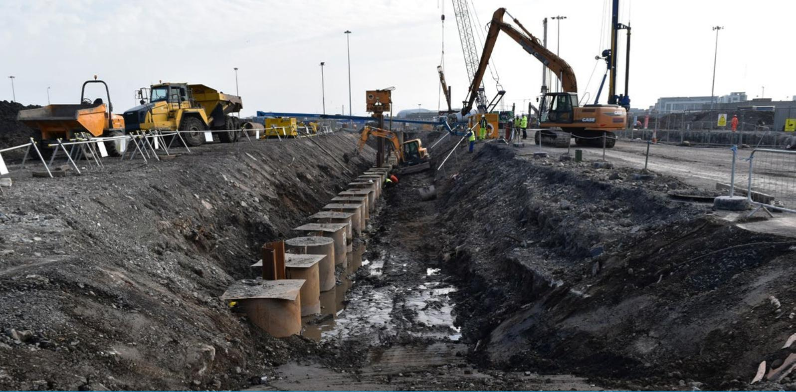
**THE ALEXANDRA BASIN REDEVELOPMENT INVOLVES THE CONSTRUCTION OF APPROXIMATELY 3KM OF QUAY WALLS, DEEPENING OF THE HARBOUR BASIN AND CHANNEL TO ACCOMMODATE LARGER SEA GOING VESSELS AS WELL AS WORKS ASSOCIATED WITH THE CONSERVATION OF THE PORT'S VICTORIAN INDUSTRIAL HERITAGE.**
