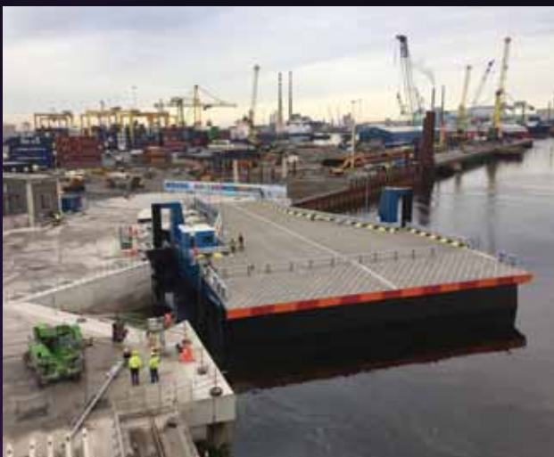
Linkspan 6 Ramp at Berth 31 in Dublin Port.
