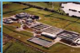
Limerick Sewerage Treatment Plant, Ireland
