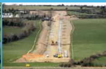
Great Island Gas Pipeline, Ireland
